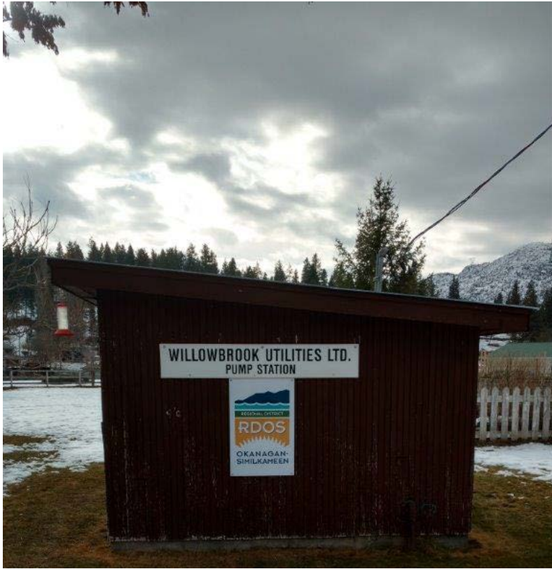
New RDOS signage at Willowbrook Utilities Pump Station.
