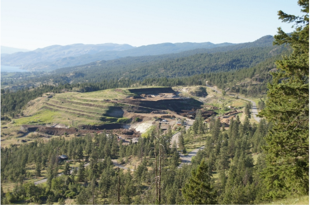
Campbell Mountain Landfill
