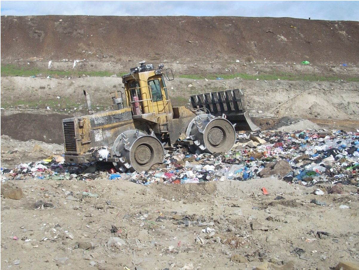
Compactor at Campbell Mountain Landfill, RDOS
